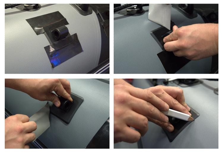
Using Gorilla Tape (or similar), tape along the pencil line to protect the outer area of the boat where the glue-on pads will not cover. Repeat for each of the pads.
